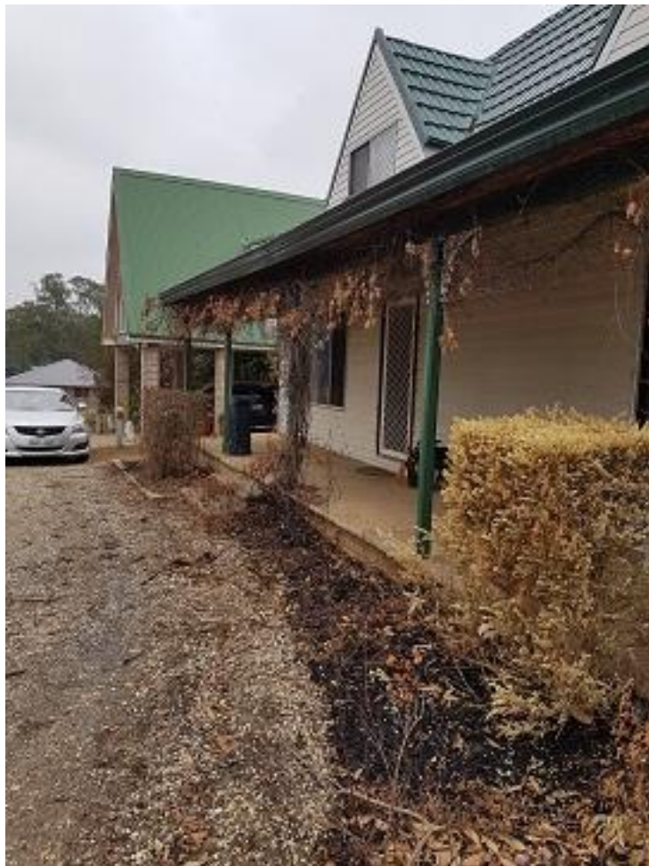
While the fire has destroyed the vine on the front verandah it has not touched the house structure.
